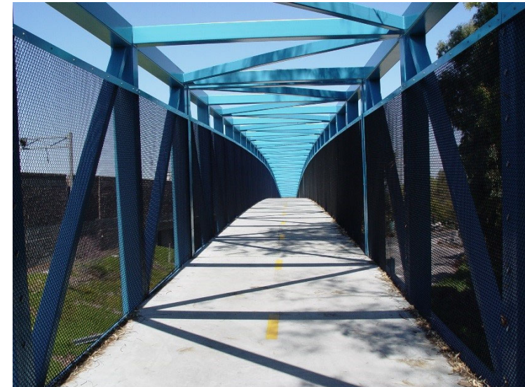
Mountain View Stevens Creek Bridge
