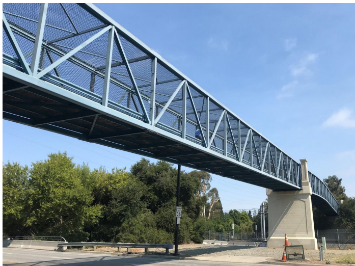
Mountain View Evelyn Avenue Bridge
