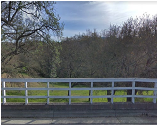
B Fence Replacement – Shire Court
