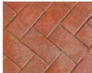
2 stamped and stained concrete slab stain color to match red bricks on the (e) sidewalk
