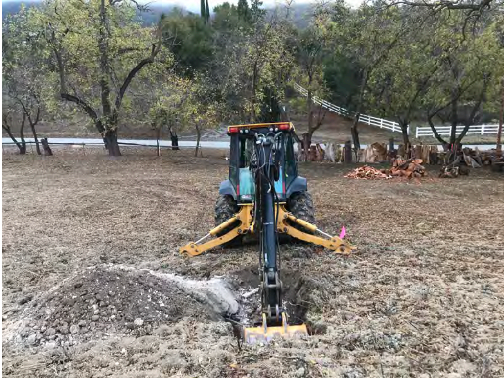
Photo 5: View of backhoe excavating Test Pit 1.
