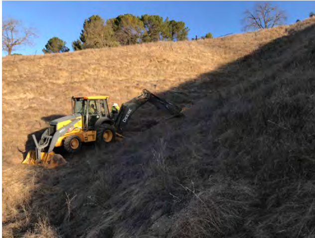
Photo 8: View of backhoe excavating Test Pit 9.
