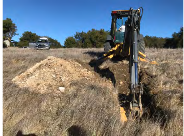
Photo 9: View of backhoe excavating Test Pit 11.
