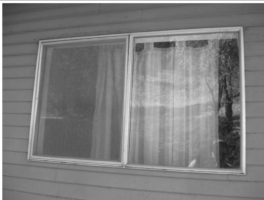
Photo 7: Detail of non-original aluminum framed window.
