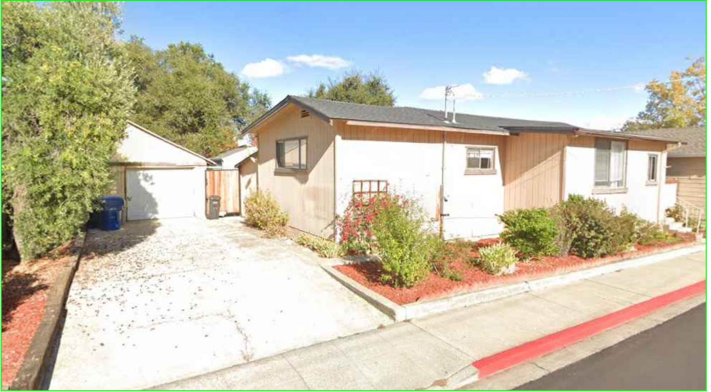
212 THURSTON ST. PROJECT SITE
