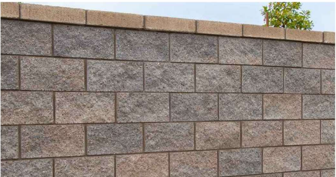
C RETAINING WALL SHALL BE VARIEGATED CMU WITH WALL CAP FROM ORCO BLOCK AND HARDSCAPE COLOR SHALL BE BORREGO SPLIT FACE ON EXPOSED SURFACE LRV SHALL BE MAX 30%
