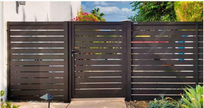
C 6' ALUMINUM PRIVACY FENCE AND GATE COLOR SHALL BE BLACK
