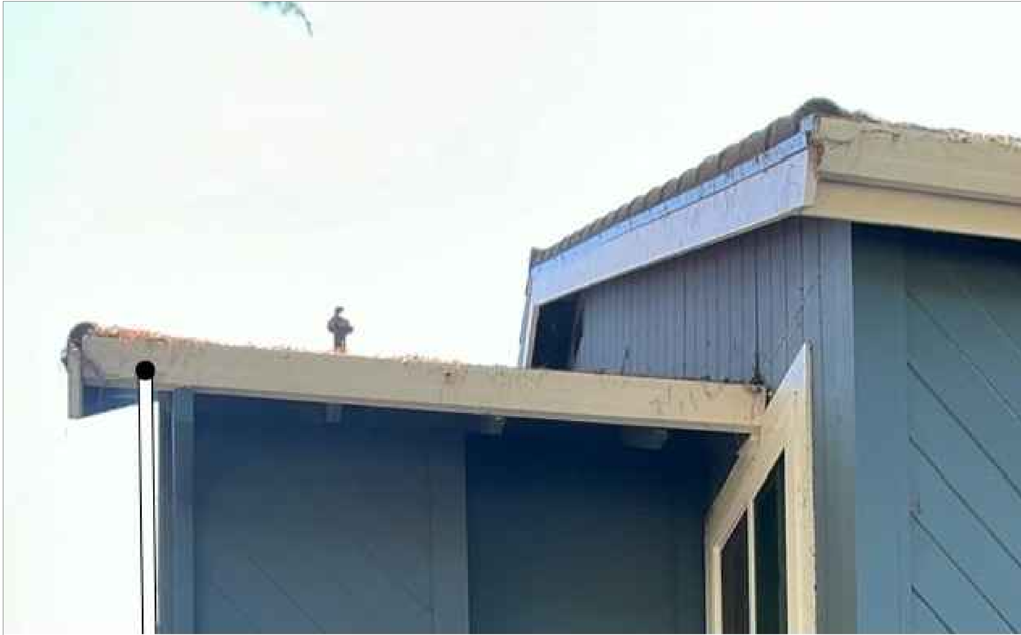
NEW FASICA & PAINT TO MATCH EXISTING
