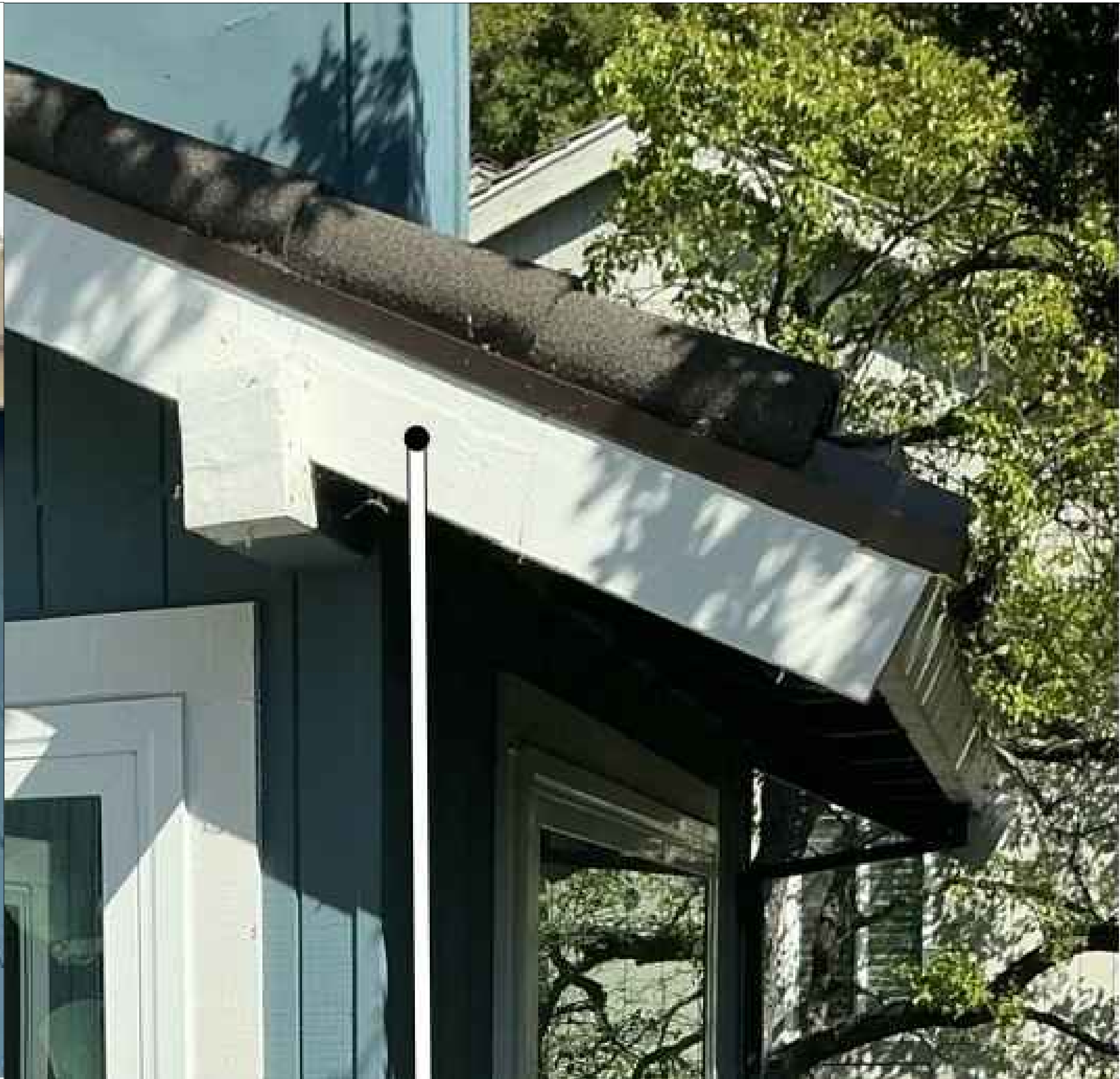
NEW DOWNSPOUT, GUTTER & PAINT TO MATCH EXISTING
