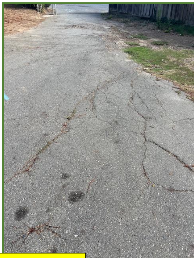
Hardscape damage due to extensive surface roots from Trees No. 947 & 948
