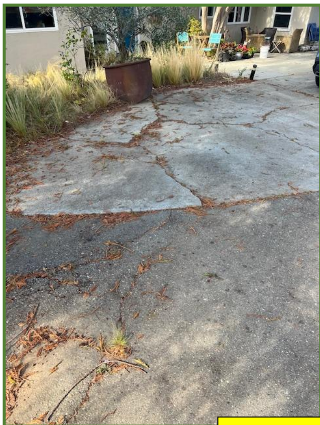
Hardscape damage due to extensive surface roots from Trees No. 947 & 948
