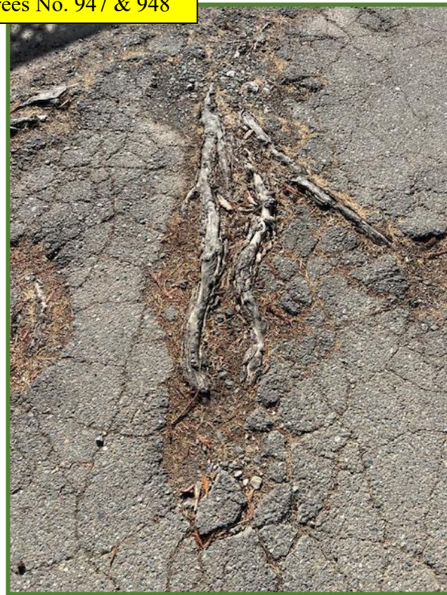
Hardscape damage due to extensive surface roots from Trees No. 947 & 948
