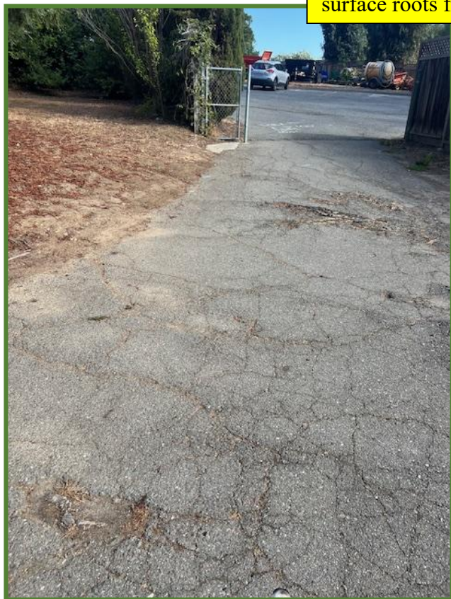
Hardscape damage due to extensive surface roots from Trees No. 947 & 948
